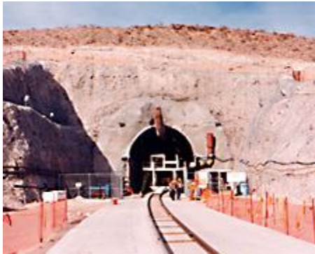
Entrance Tunnel at Yucca Mountain
